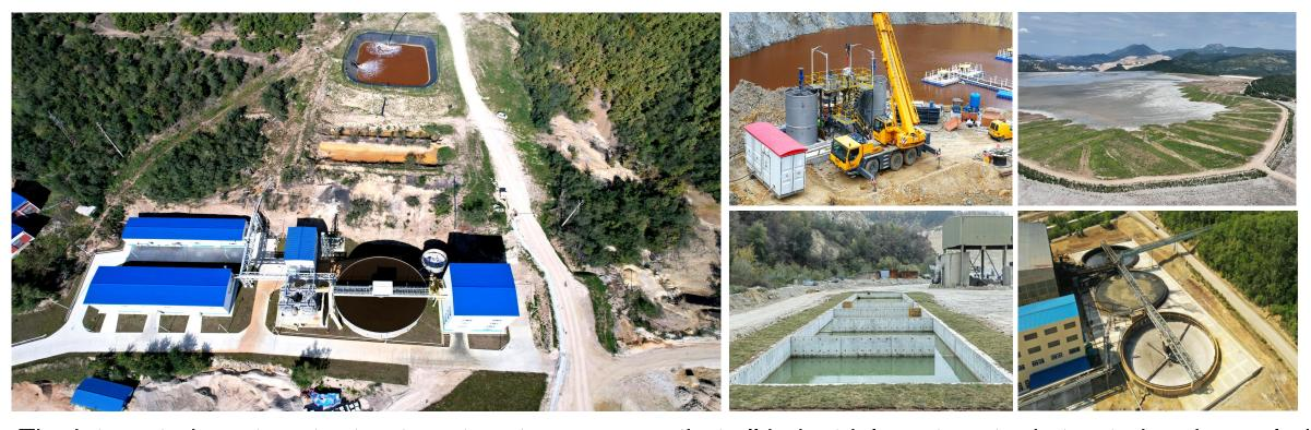
The integrated wastewater treatment systems ensure that all industrial wastewater is treated and recycled to use again. Mine pit wastewater is injected into the tailings pond, neutralized and precipitated, and then reused.
