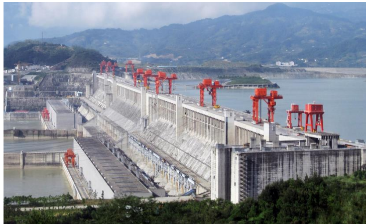
Figure 4 Hydroelectric power plants [12]
