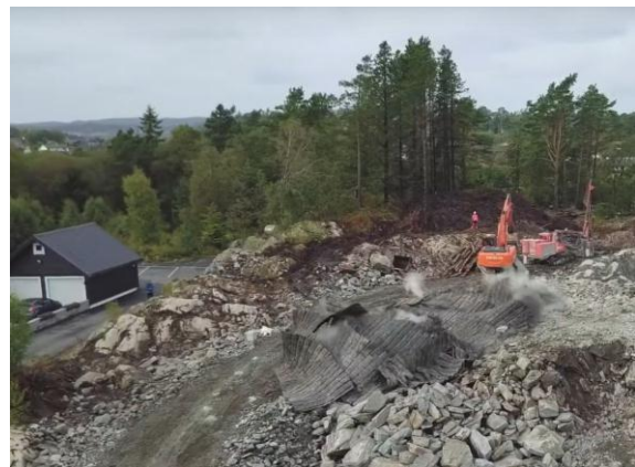
Figure 5 Initiation of blasting charges covered with blasting mats in urban blasting [14]
