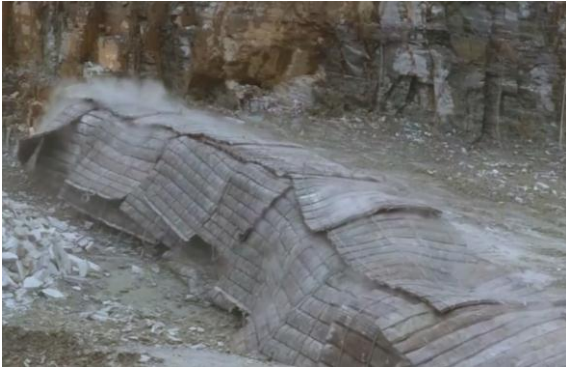
Figure 6 Blast field covered with blasting mats in quarry rock blasting [14]
