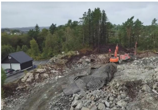
Figure 4 Blast field covered with blasting mats in urban blasting [14]
